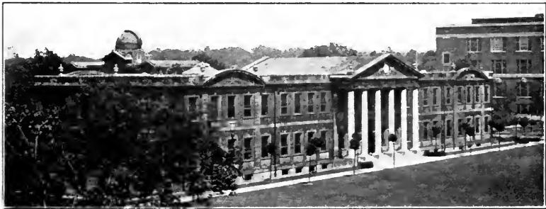
Upper Photo—Nela Operating Building.
